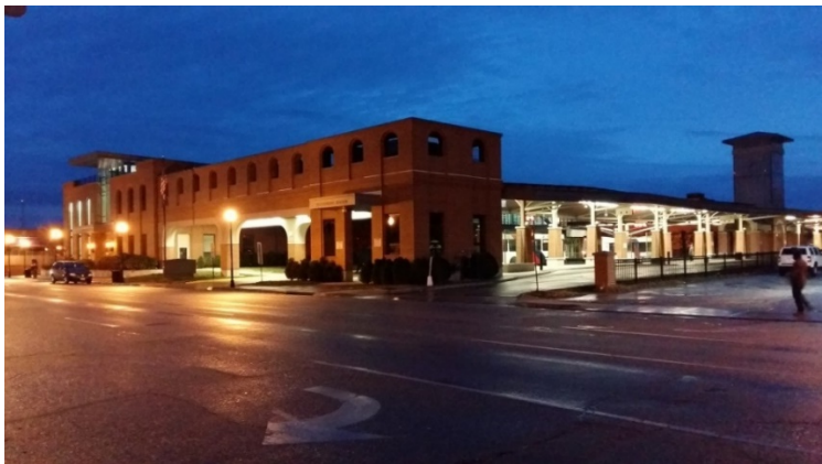
Figure 3-7: Petersburg Multi-Modal Station
