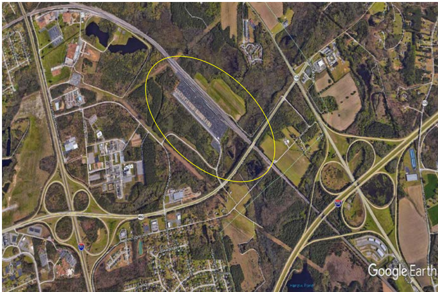
Figure 3-22: NS Automobile Distribution Facility
