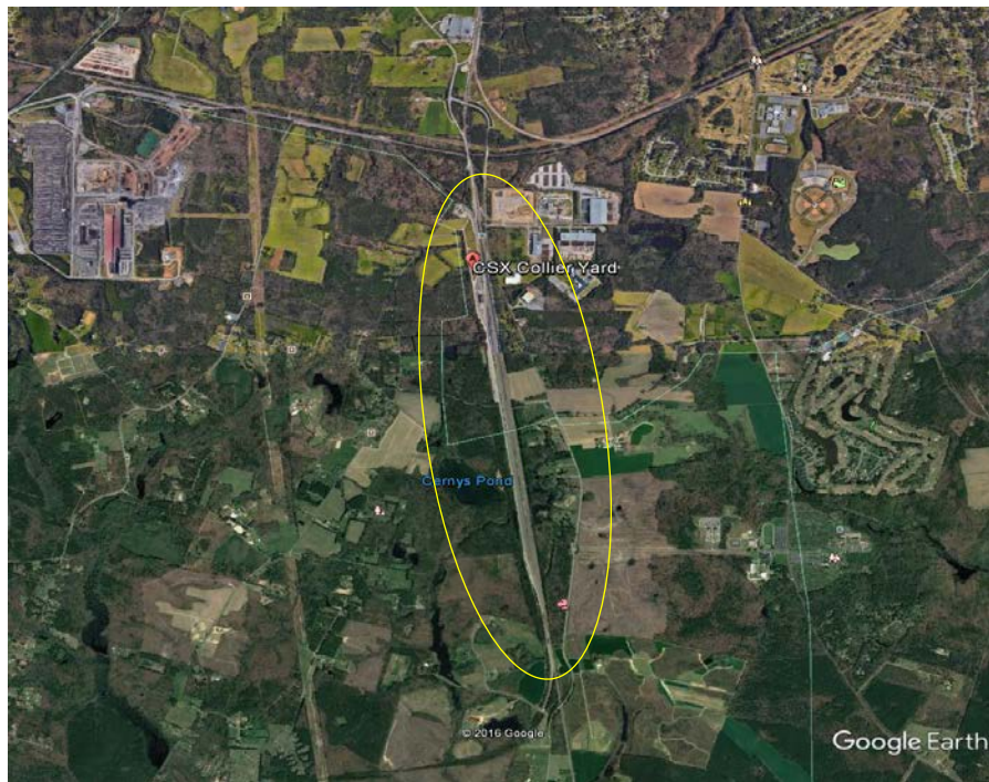
Figure 3-23: CSX Collier Yard
