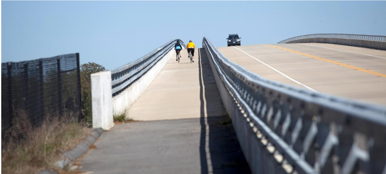
The Judith Stewart Dresser Memorial Bridge, which carries Route 5 and the Virginia Capital Trail over the Chickahominy River, includes a 10' shared-use path (separated by a barrier)
