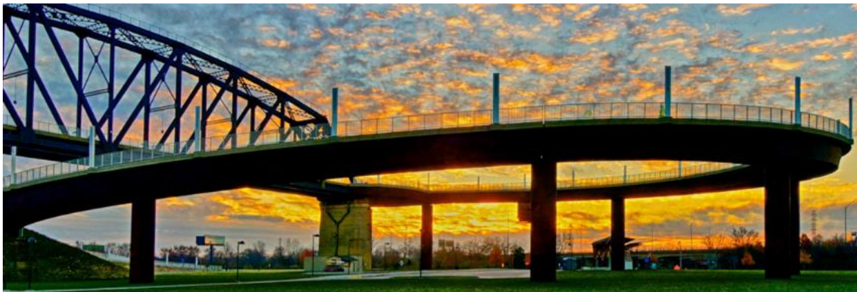
Big Four Bridge: Louisville, Kentucky. Source: Louisville Waterfront
