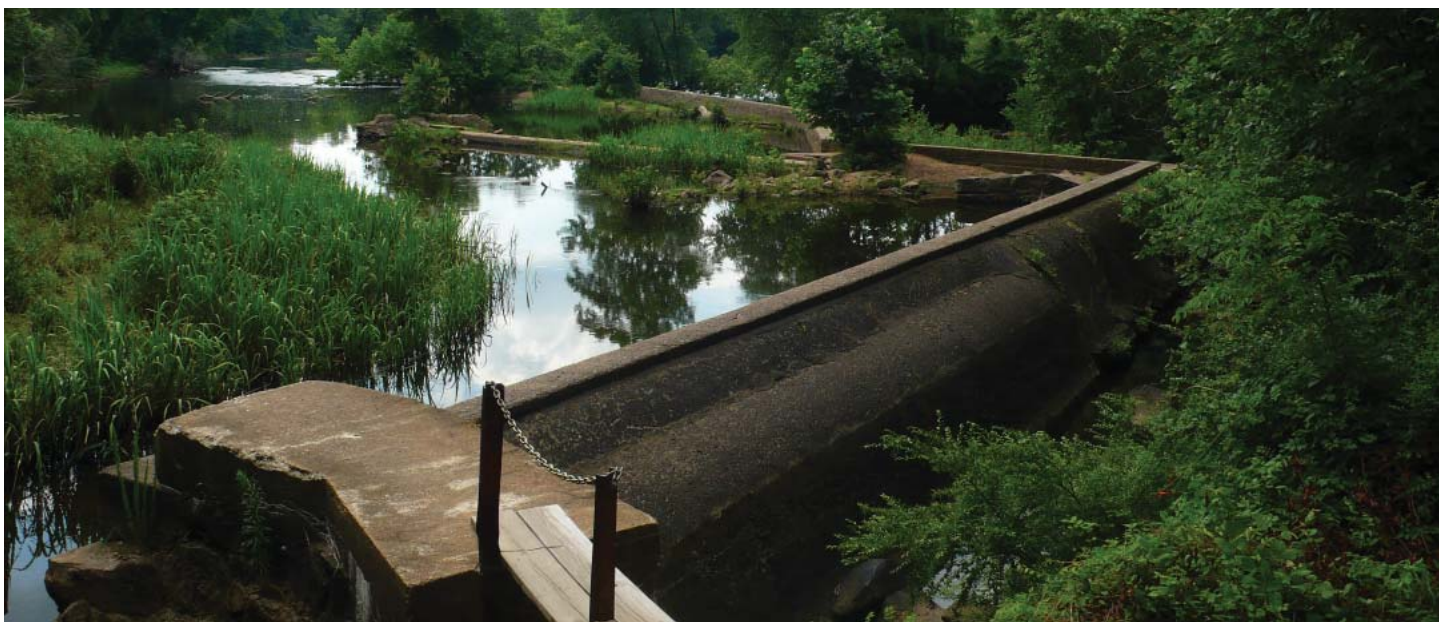
Historic Abutment Dam
