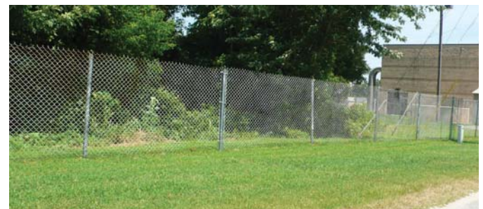
Fence at Wastewater Treatment plant (from inside facility)
