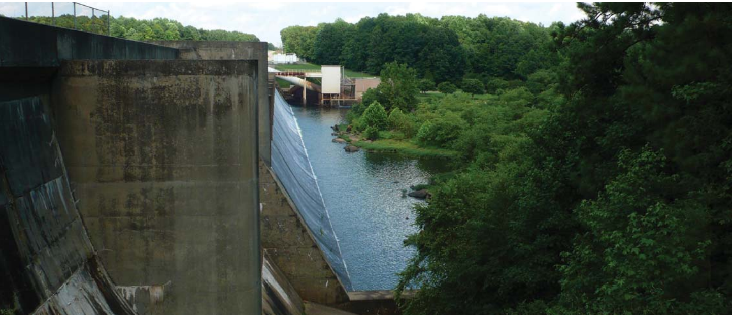
Dam at Lake Chesdin
