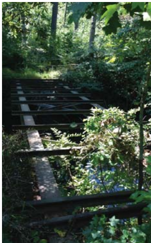
Existing bridge frame
