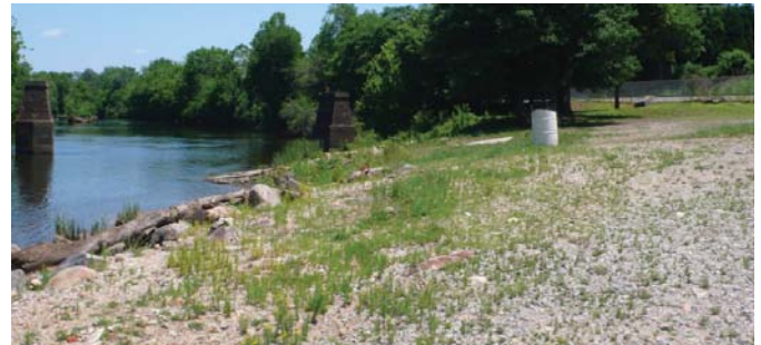
Existing conditions along edge of river
