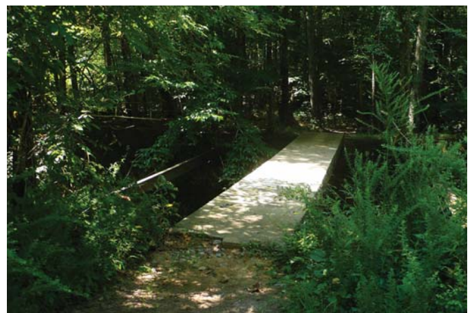
Existing footbridge across canal
