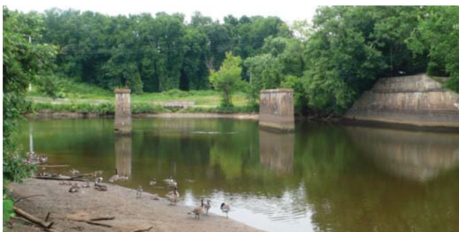
Existing bridge abutments
